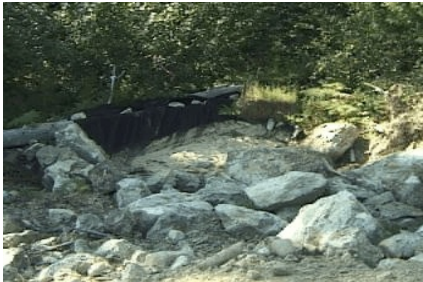
Photo 2 – Filter fabric at culvert outlet
